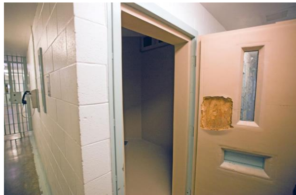
Existing Safety Cell (under-repair).
