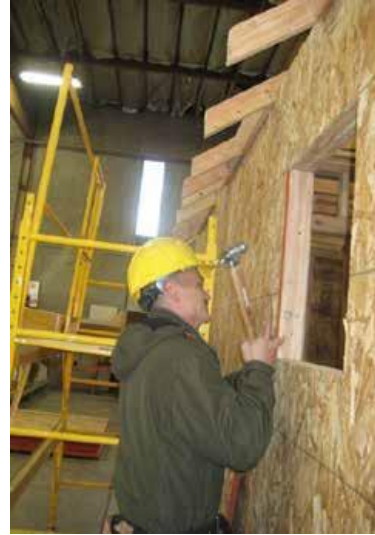
The Sheriff's Home Detention Program and Probation's Adult Day Reporting Centers have 50 work experience training slots available to provide GED testing and construction trade classes with links to over 20 unions for job placement
