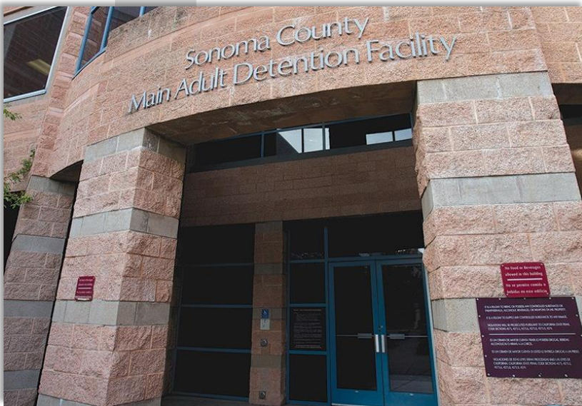
Main Adult Detention Facility
