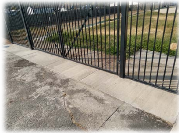
Poured concrete bases for fencing at the Twain Harte and Columbia pools
