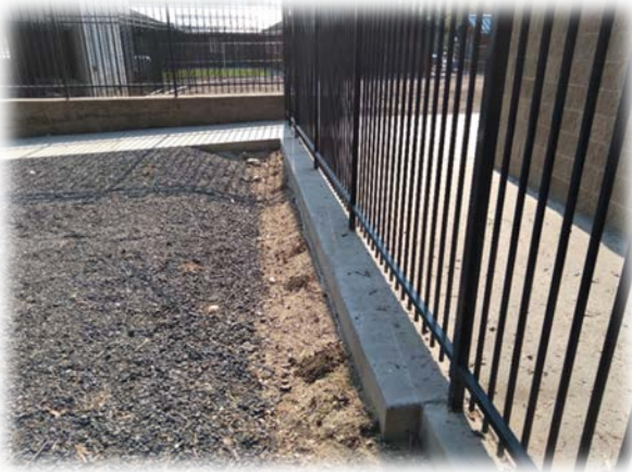
Poured concrete bases for fencing at the Twain Harte and Columbia pools
