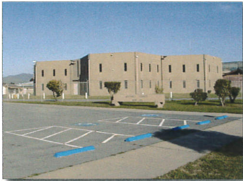
The Monterey County Main Jail.
