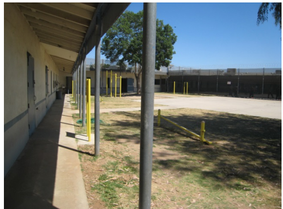
Housing C – Exterior Walkway
