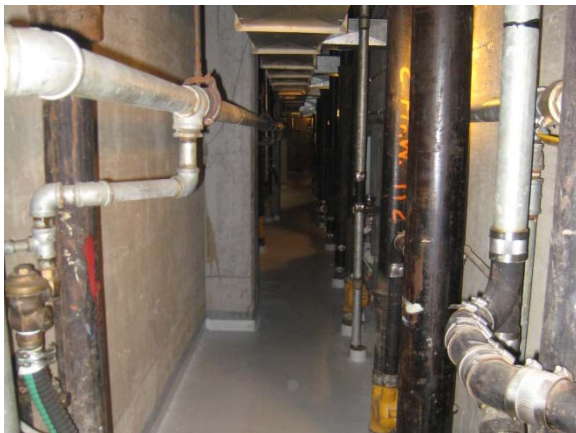
Housing Plumbing Chase
