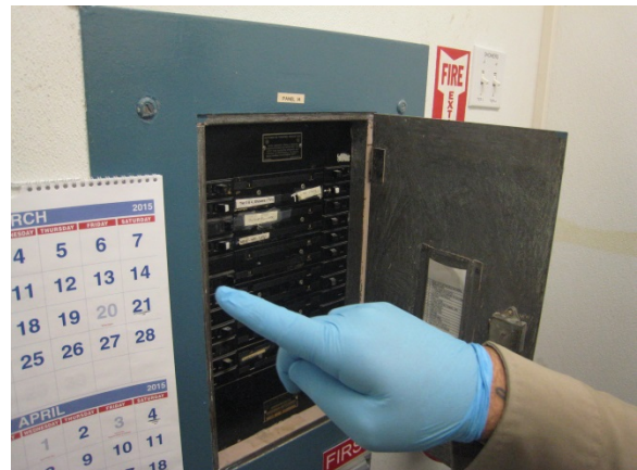
Housing Door Control Panel
