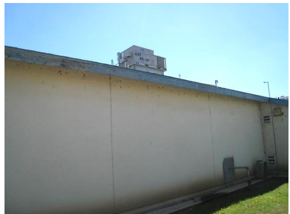
Housing A – Exterior / Roof-top Mechanical
