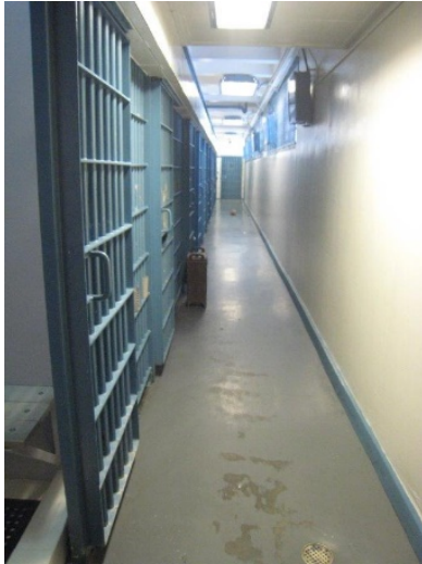
Main Jail Typical Housing Unit
