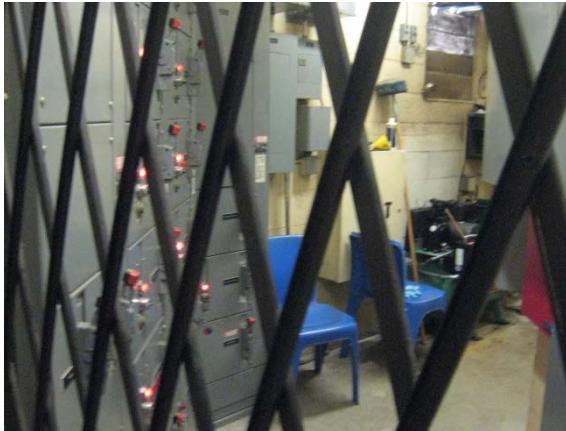
Housing Unit Electrical Room
