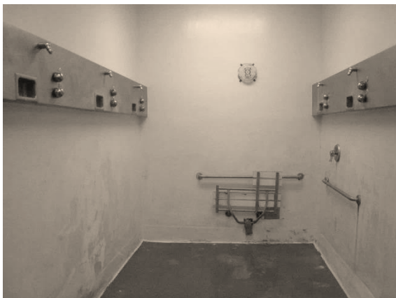
Housing B – Shower Room
