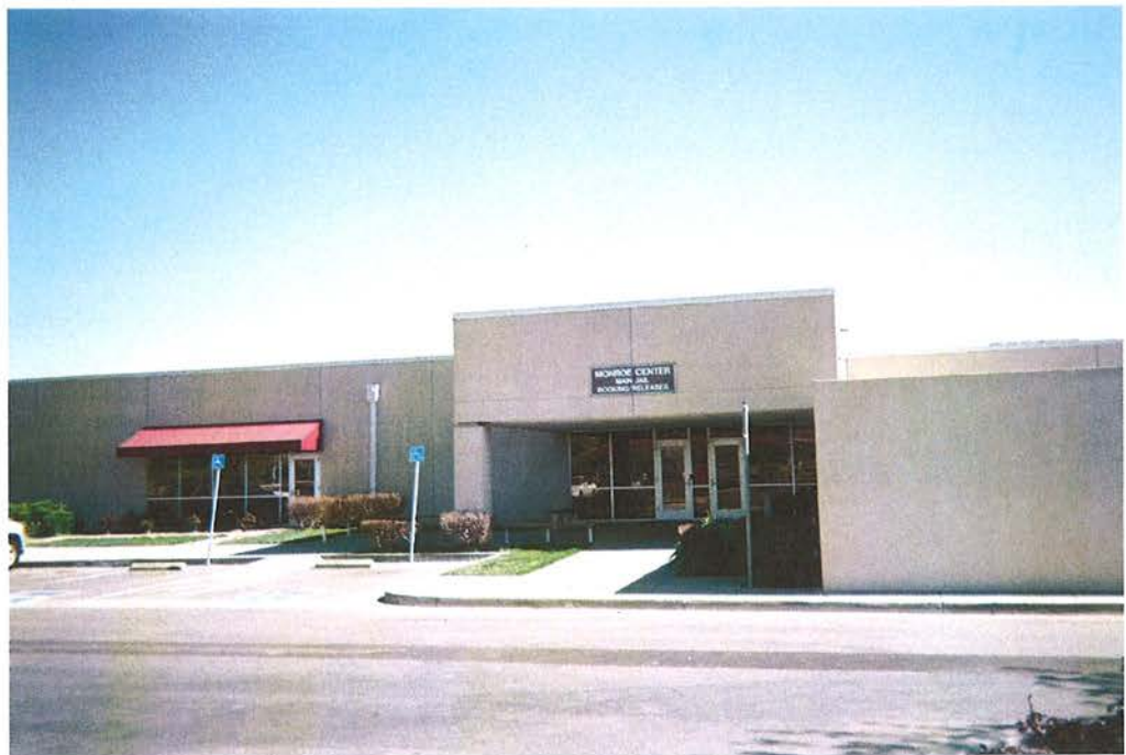
Yolo County Monroe Center Main Jail 2420 East Gibson Road, Woodland, CA 95776
